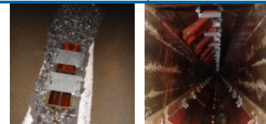
Completely evacuated flushing channel
