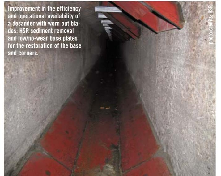
Improvement in the efficiency and operational availability of a desander with worn out blades: HSR sediment removal and low/no-wear base plates for the restoration of the base and corners.
